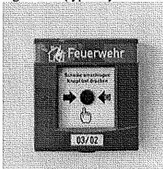
A call point from a conventional fire alarm system
